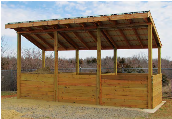
Photograph 2. A permanent three-bin wooden mortality composting structure.
